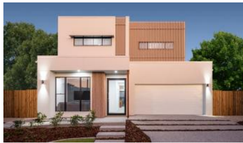
48 Hart Crescent, Bells Creek
